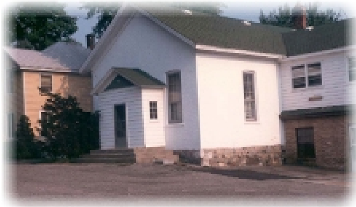
Former Walker Township Hall Leonard St & Covell Ave.
